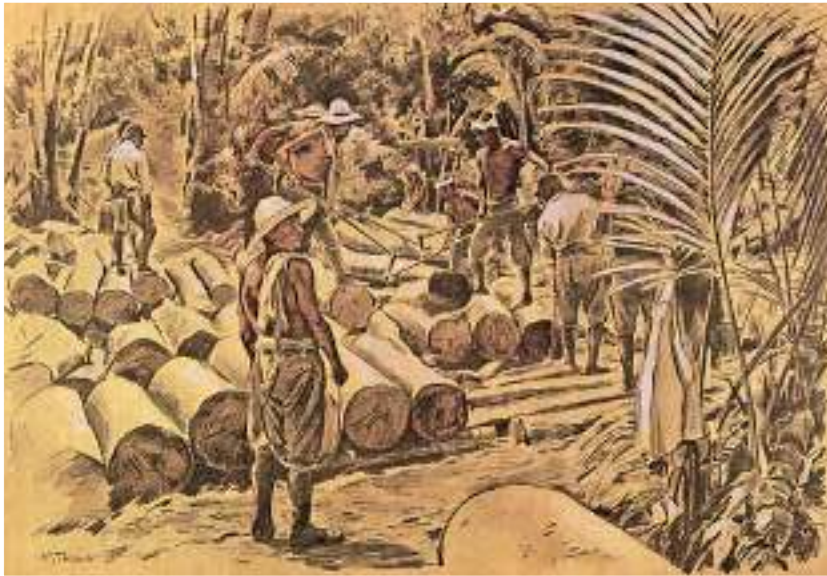
Japanese troops and local laborers cutting hardwood logs for revetting gun positions. Local laborers were used extensively for constructing support facilities, wood-cutting, and transporting materials, but the troops themselves constructed most of the fighting positions and defenses. (Original painting by Manjiro Teracuchi)
