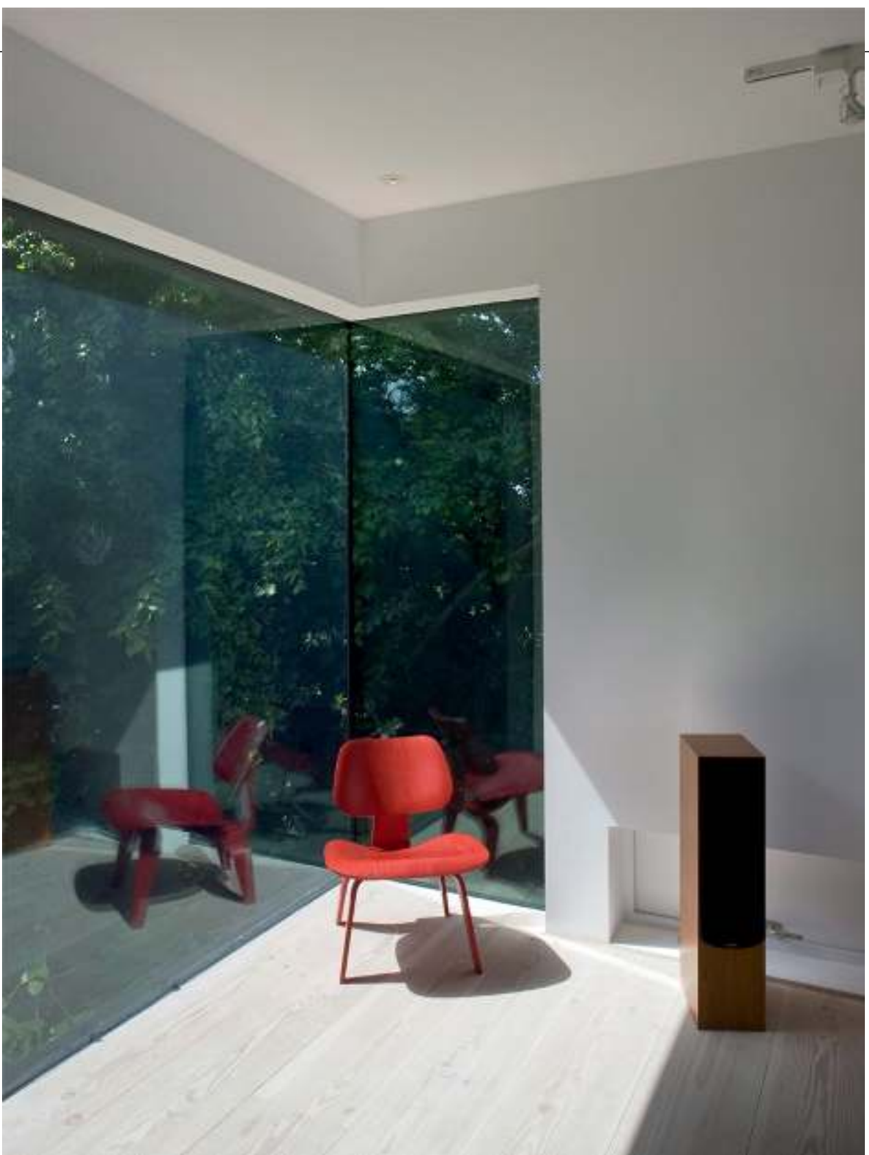
Glazed corner windows, made from fixed double-glazing, afford woodland views (© Morley Von Sternberg)
